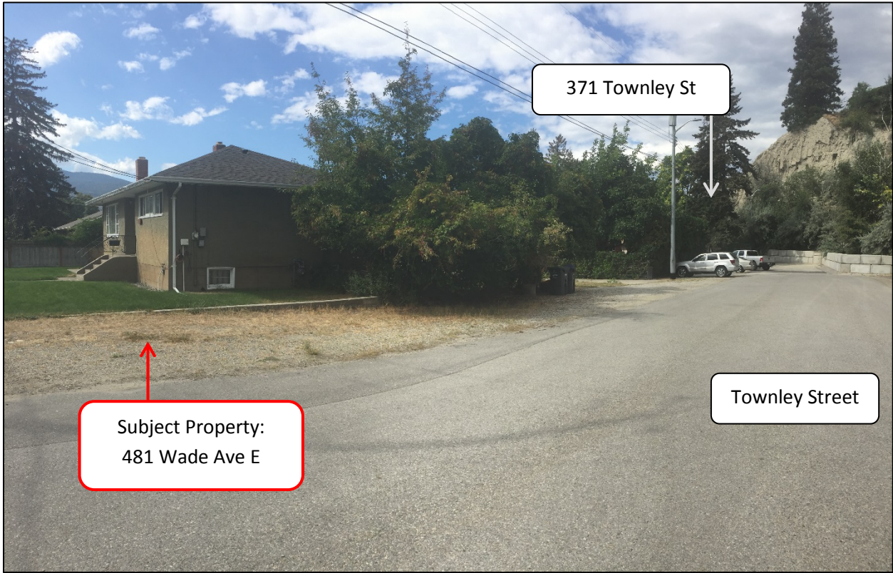
Figure 8 – Looking at 481 Wade Ave E from Townley Street
