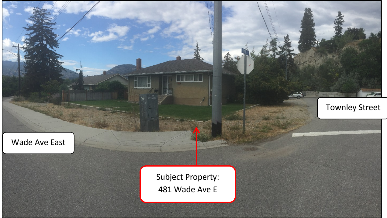
Figure 4 – Looking toward front of 481 Wade Avenue East from corner of Wade Ave and Townley Street
